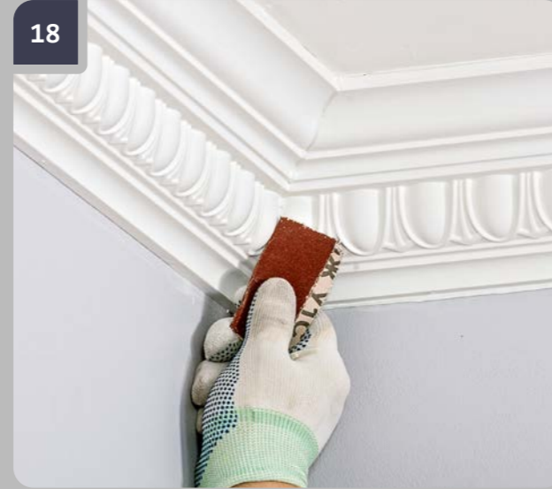
18 After 3 hours treat the joints with fine grain abrasive paper.
