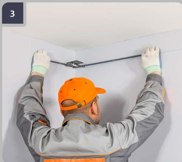
3 Using the adjustable square measure the angles of the room.
