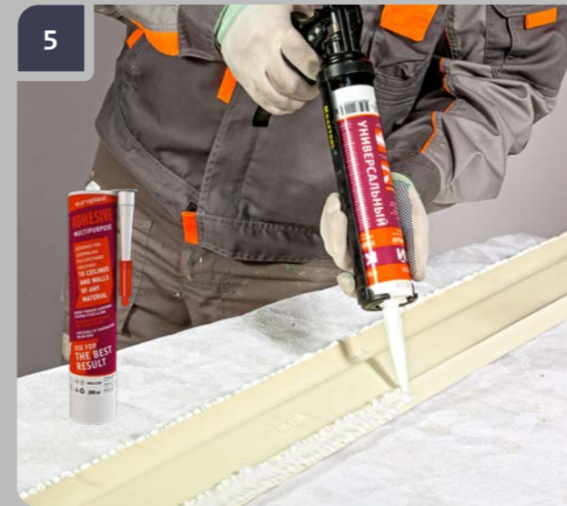
5 Apply evenly on the mounting surface Europlast multipurpose adhesive along the whole length. The thickness of the applied adhesive should be 3-5 mm.
