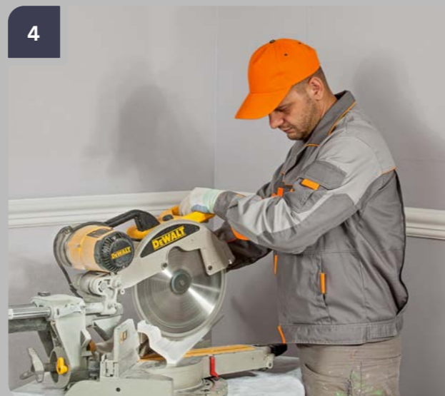
4 Using a mitre saw, cut out the element to the appropriate angle. In a room with 90° angles a mitre box or a handsaw can be used.
