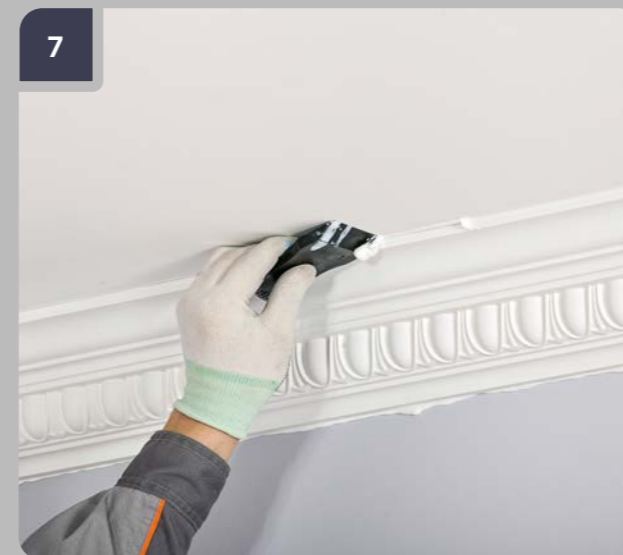
7 Immediately after gluing remove the excess of Adhesive with a spatula.
