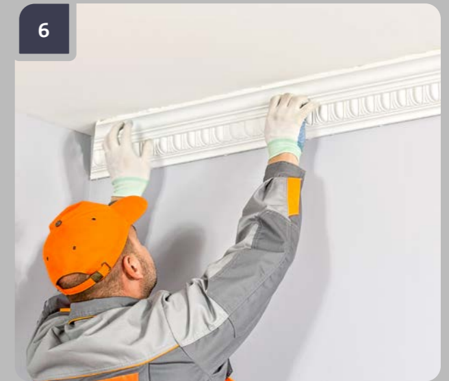
6 Attach the item to the place of installation, using as benchmarks the previously made marks on the wall. Push the entire length of the item so the adhesive exudes from the entire plane.
