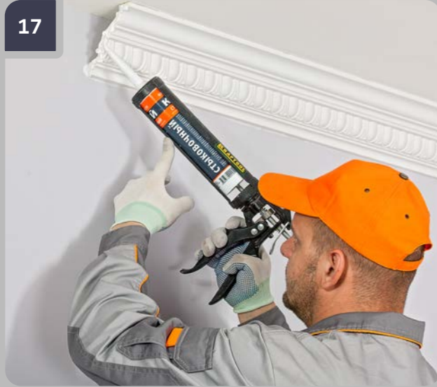
17 Continue the process of installation of the next cornice.
