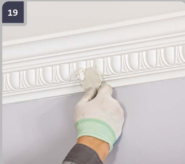
19 Fill the treated area with fine-grained, water-soluble filler for interior works, repeat Step #18 if needed, until you get a flat surface.
