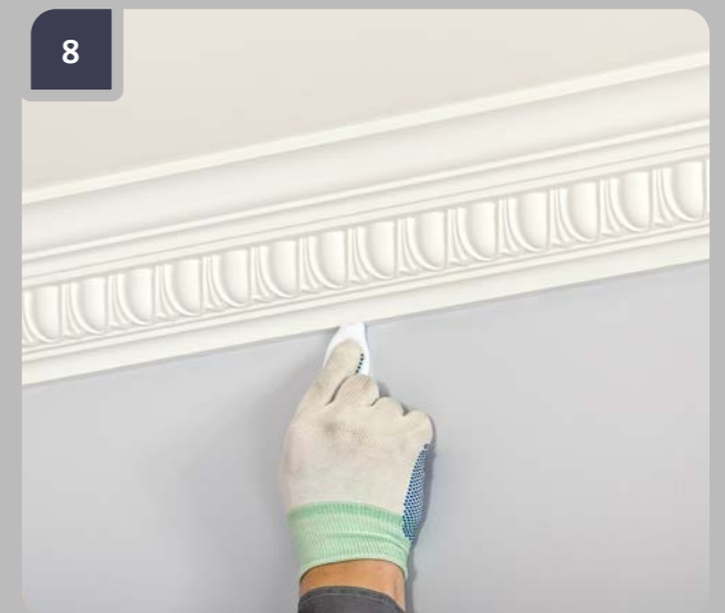
8 When using Assembly Adhesive, remove the remaining excess of adhesive by wiping the areas with a cloth dampened with water; use acetone if Multipurpose adhesive is used.
