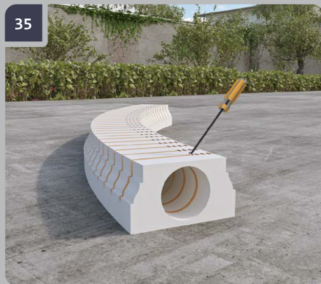
35 Remove the staples 24 hours later.
