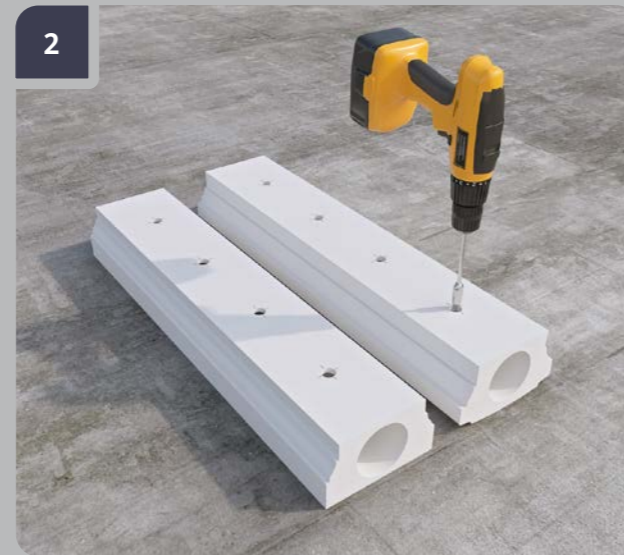
2 Use the Ø20 mm drill bit.
