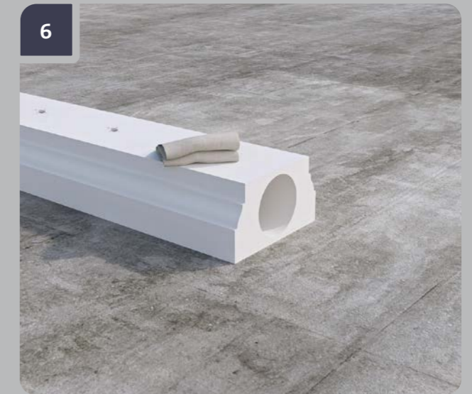
6 Clean out the dust and dirt from the ends of the adjoining items with a wet cloth.
