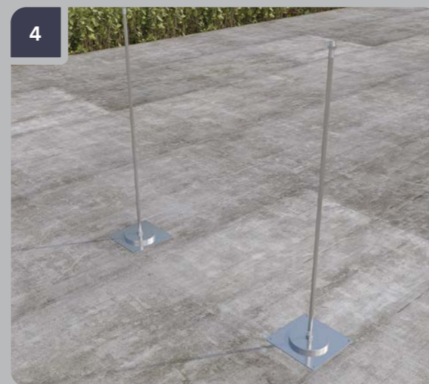
4 Fasten the flanges to the surface with the help of anchor bolts.
