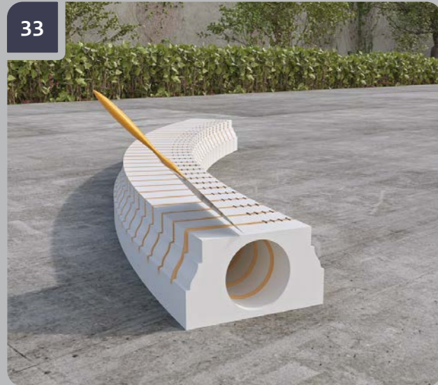
33 Remove excessive glue with a scraper.
