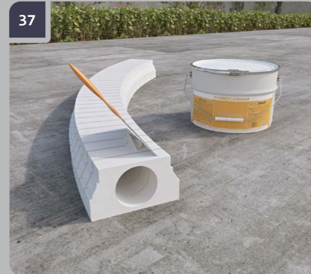
37 Fill the cuts with putty.
