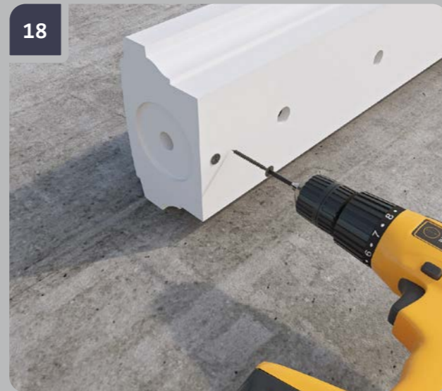
18 Screw the plug to the handrail using self-tapping screws.
