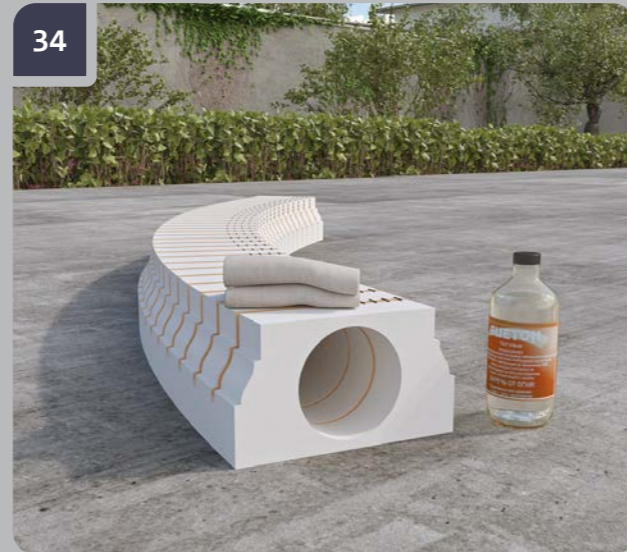
34 Remove excessive glue with a cloth dampened with acetone.
