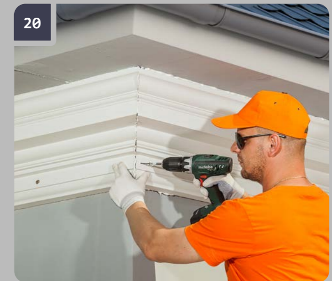
20 Attach the joint with self-tapping screws.
