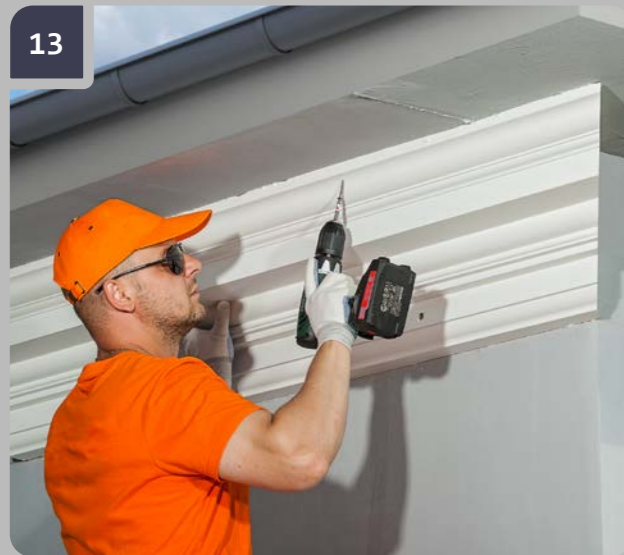
13 With the screw gun and a self-tapping screw pull the upper part of the item and sink the screw's top 2 mm into it.
