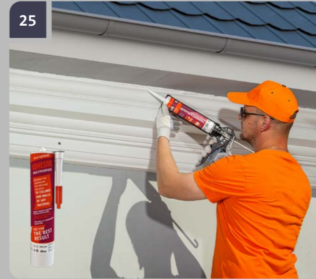
In places where an item abuts the surface and no adhesive has exuded from the joint, fill the gaps with more adhesive.
