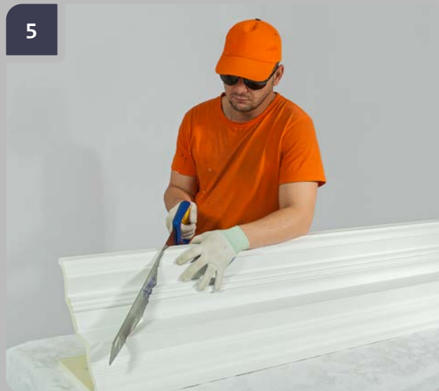
5 Finish the cut with a hand saw.
