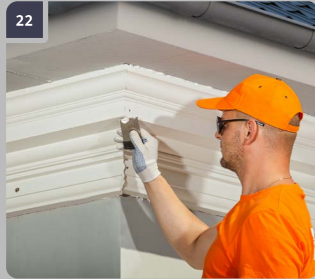
Remove excess adhesive with a palette knife immediately after gluing.
