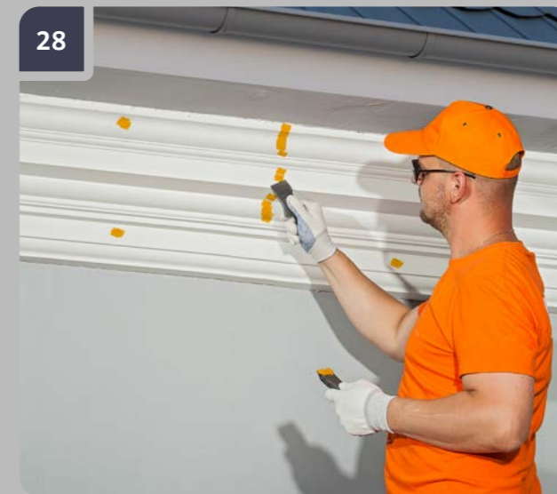
Apply putty to the treated spots and over the heads of screws — use automotive putty.
