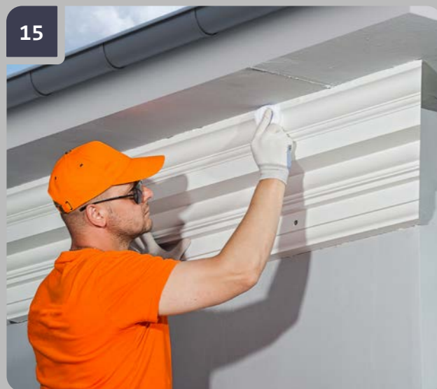
15 If necessary, rub the spots where the item touches the surface with an acetone-soaked cloth.
