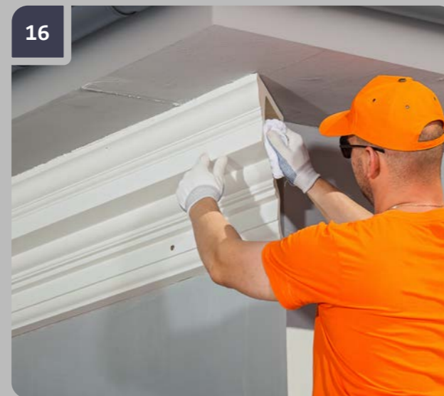
16 Use a moistened cloth to clean the butt ends of the adjoining items from dust and other dirt.
