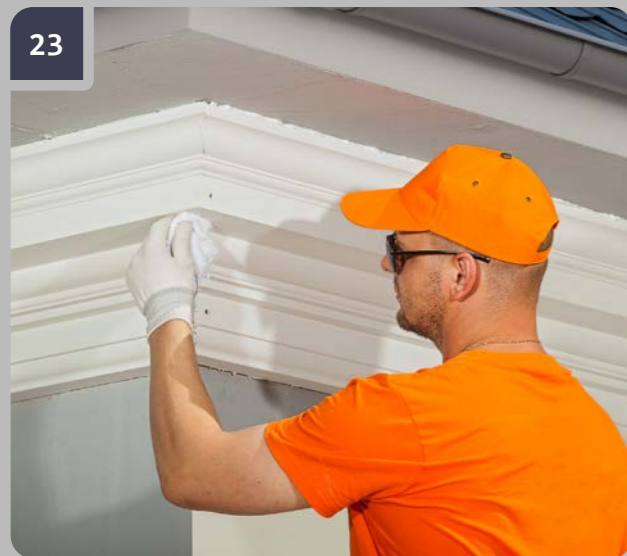
Rub the joint with an acetone-soaked cloth.
