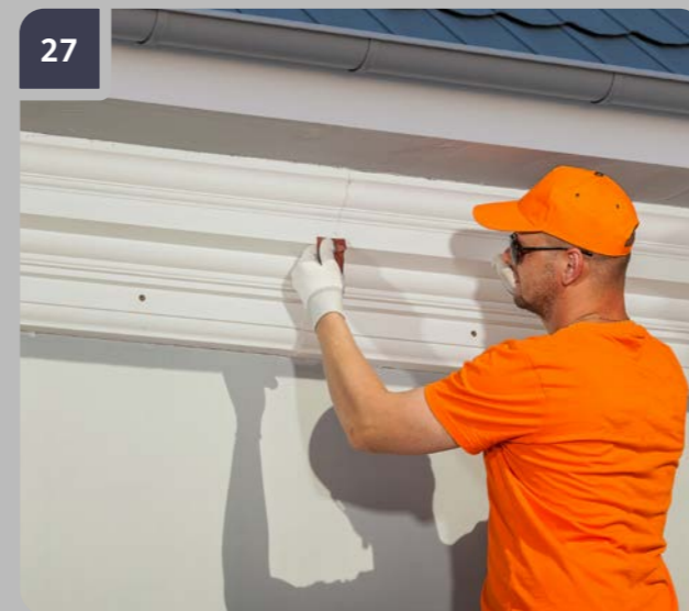
Wait 3 hours and apply soft sand paper to the joints for an even surface.
