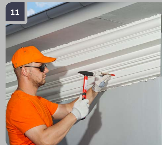
11 Fix the item in place with impact anchors.
