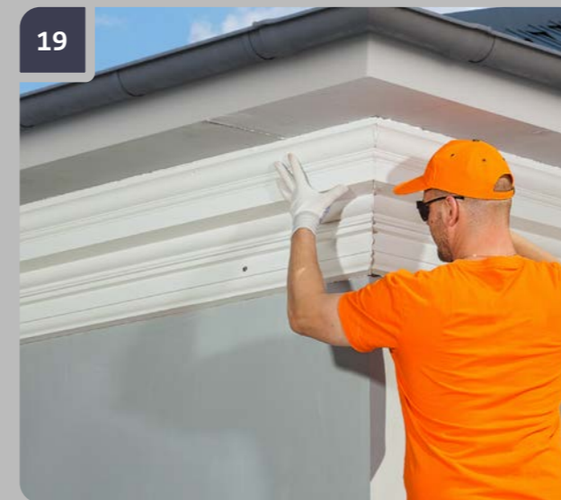
19 Attach the item to the mounting spot. Press along the entire length hard enough to make adhesive exude from the joint. Sliding the item along the wall, press it against the neighbouring item so that adhesive exudes from the joint.
