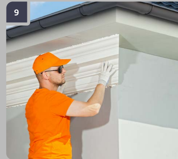
9 Place the item to the mounting spot, according to the markings on the wall. Press the item along the entire length hard enough to make the adhesive exude from the joint.
