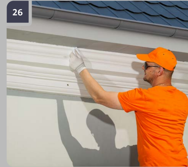
Use acetone and cloth to remove extra adhesive.
