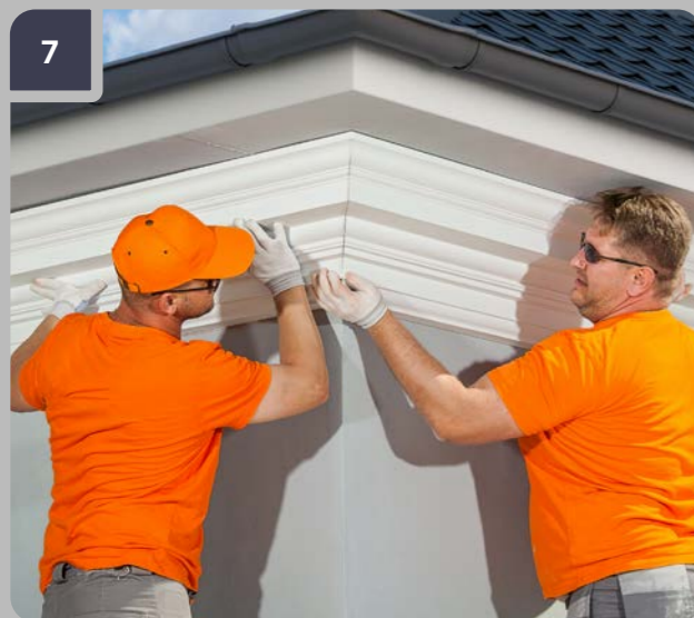
7 Check that the item's pattern and profile match.
