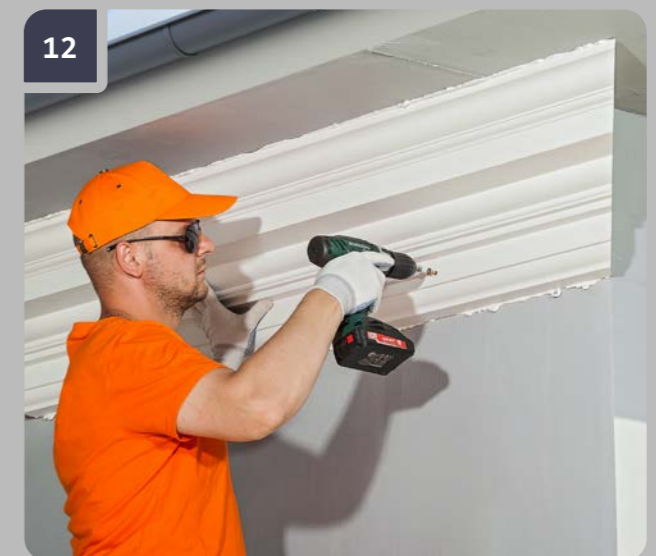
12 Use a screw gun to drive the impact anchors' heads into the item – 2 mm deep.
